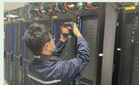
▲ Thermal imaging scanning was carried out in Daoxianghu machine room in Beijing. (Photo provided by the Data Center)
