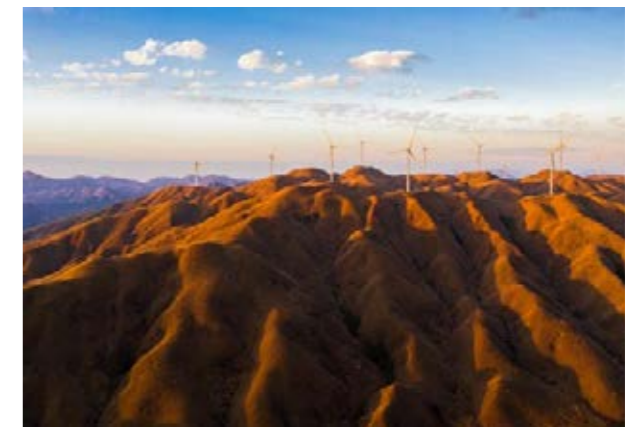
▶ Guangxi Branch supported the construction of wind farm projects. (Photo provided by Guangxi Branch)
