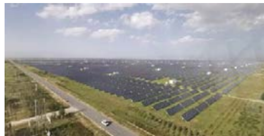
▲ Qinghai Branch supported the construction of new energy base projects. (Photo provided by Qinghai Branch)
