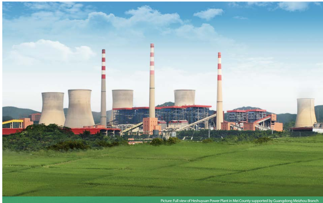
Picture: Full view of Heshuyuan Power Plant in Mei County supported by Guangdong Meizhou Branch
