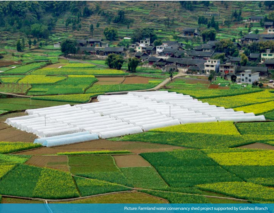
Picture: Farmland water conservancy shed project supported by Guizhou Branch
