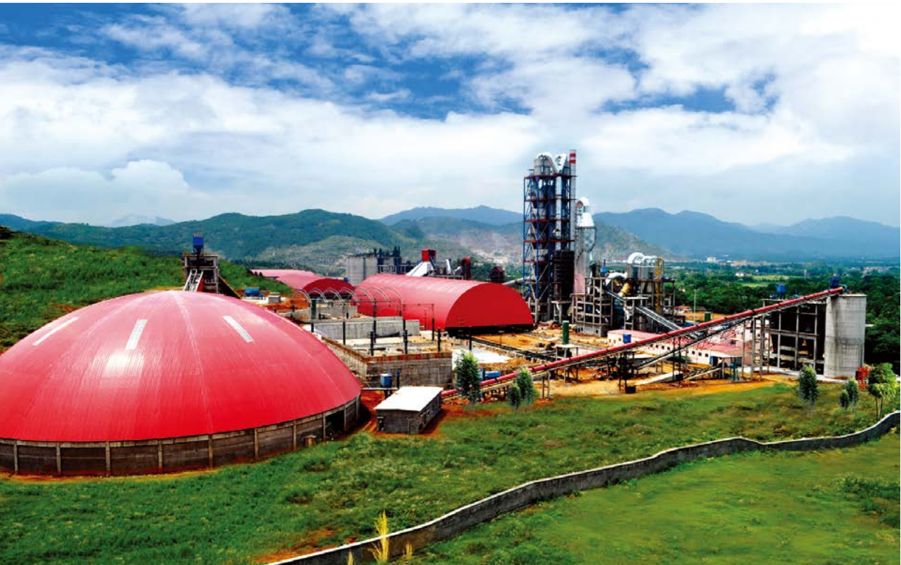
Picture: Full view of the factory buildings of Hongshi Cement Group after energy-saving technological transformation under the support of Zhejiang Branch
