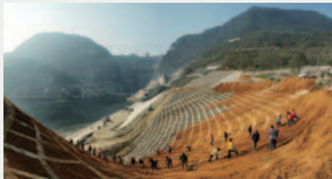
贵州分行支持“西电东送”工程构皮滩水电站 Guizhou Branch supported Goupitan Hydropower Station of “West-East Power Transfer” Project
