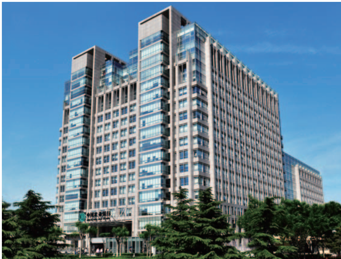
北京建国门内大街69号农业银行总行办公大楼 Office Building of Agricultural Bank of China H.O., 69 Jianguomennei Avenue, Beijing
