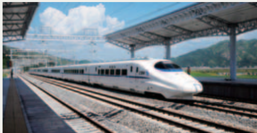
浙江分行支持甬台温铁路建设 Zhejiang Branch supported the construction of Ningbo-Taizhou-Wenzhou Railway
