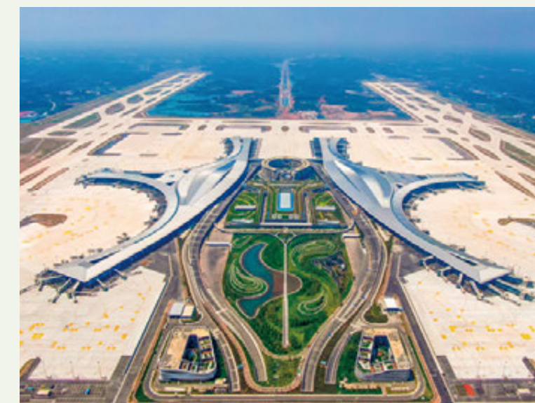
▲ ABC Sichuan Branch supports the construction of Chengdu Tianfu International Airport. (Photo credit: ABC Sichuan Branch)
