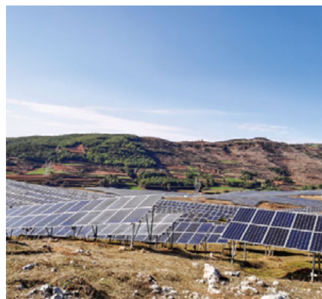
ABC Guizhou Branch supports the construction of the photovoltaic power station project. (Photo credit: ABC Guizhou Branch)
