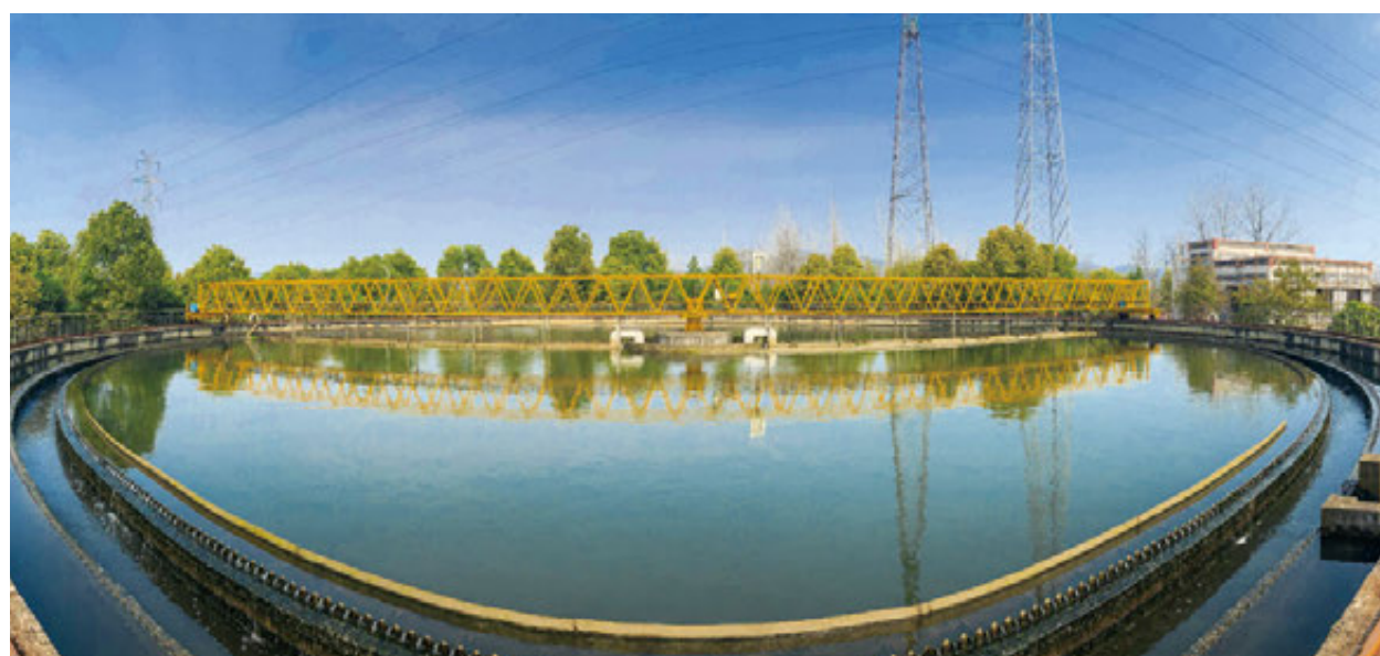
ABC Tianjin Branch supports the upgrading and renovation of sewage treatment facilities. (Photo credit: ABC Tianjin Branch)
