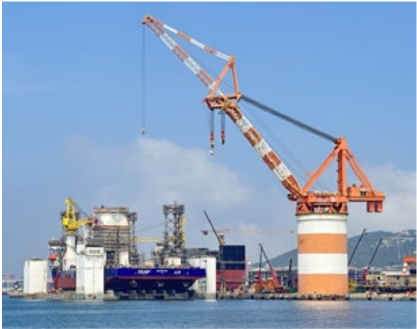
ABC Financial Leasing actively carried out direct leasing business for an offshore wind power installation vessel. (Photo provided by ABC Financial Leasing)
