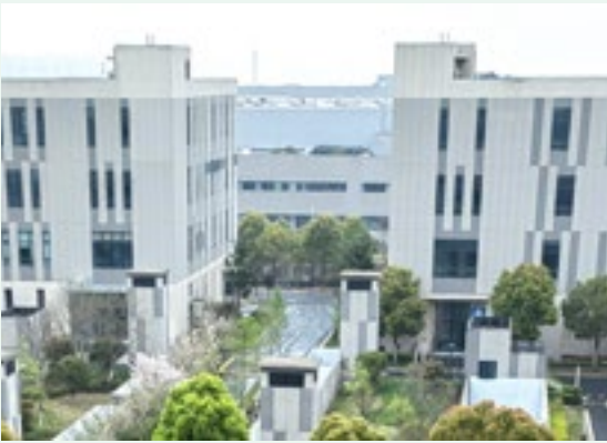
▲ The Bank’s data centers are accelerating their green and low-carbon transition. (Photo provided by the Data Center)
