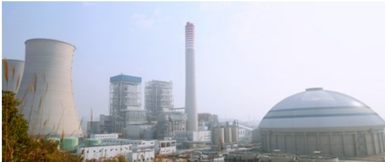
▲ Guangxi Branch supported the construction of a clean and efficient coal utilization project. (Photo provided by Guangxi Branch)
