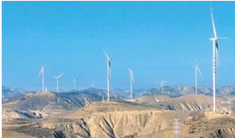
▲ Shaanxi Branch supported the construction of Shaanxi Zichang Lijiacha wind power project. (Photo provided by Shaanxi Branch)
