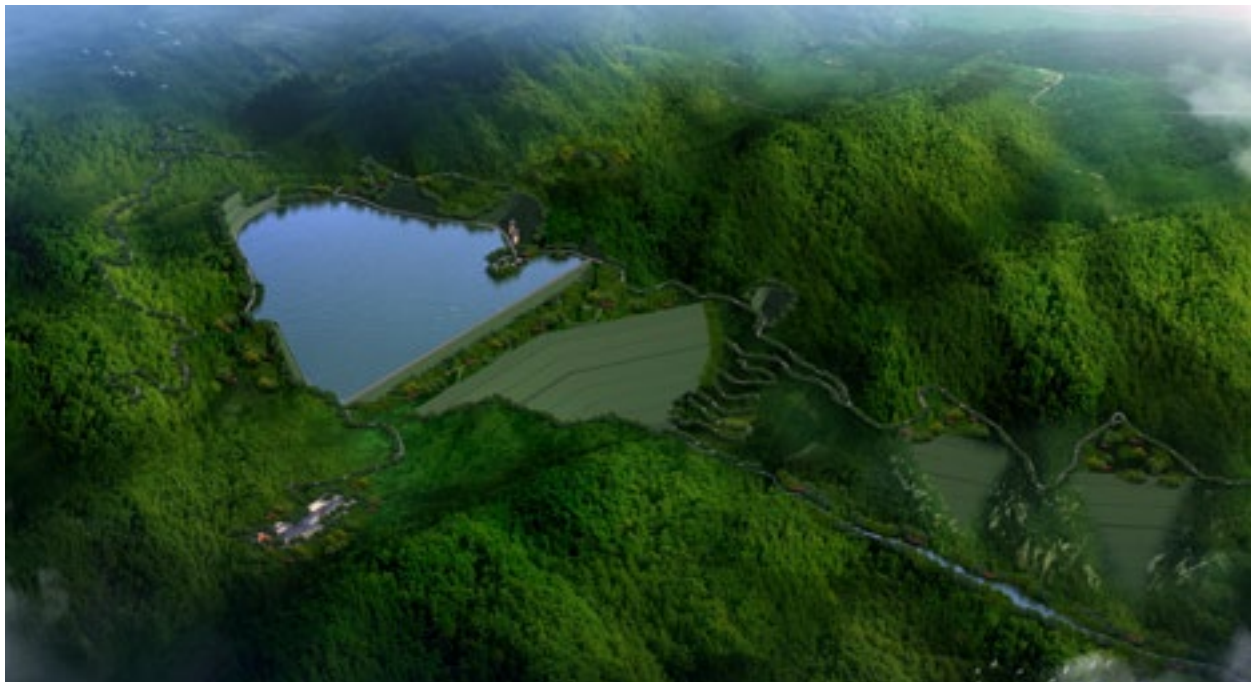
▲ Henan Branch supported a regional pumped storage power station project. (Photo provided by Henan Branch)
